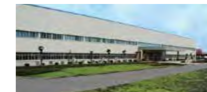
FG.L.S Electric Co., Ltd. (China)
